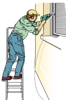
Figure 2a Incorrect - steps side-on to work activity
